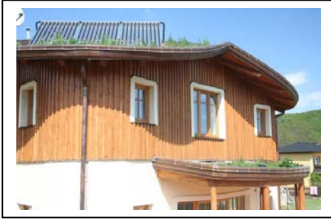
Pic 7 - House facade in May. As you can see from the size of the shadow, the overlapping roof shades the southern and western walls keeping the interior free from overheating. The wooden facade and the roof are aerated. The solar collectors are used for heating water.
