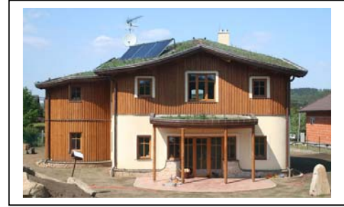
Pic 8 - Southern facade of the family house. Enclosure walls are made of 24 cm (9.5 in) thick thermal insulation bricks. Walls, roof and ground floor are insulated with mineral wool 20, 24 and 14cm thick (7.9, 9.5 and 5.5). Overall heat loss is 8.6 kW. Heating source is a gas furnace - 11 kW.
