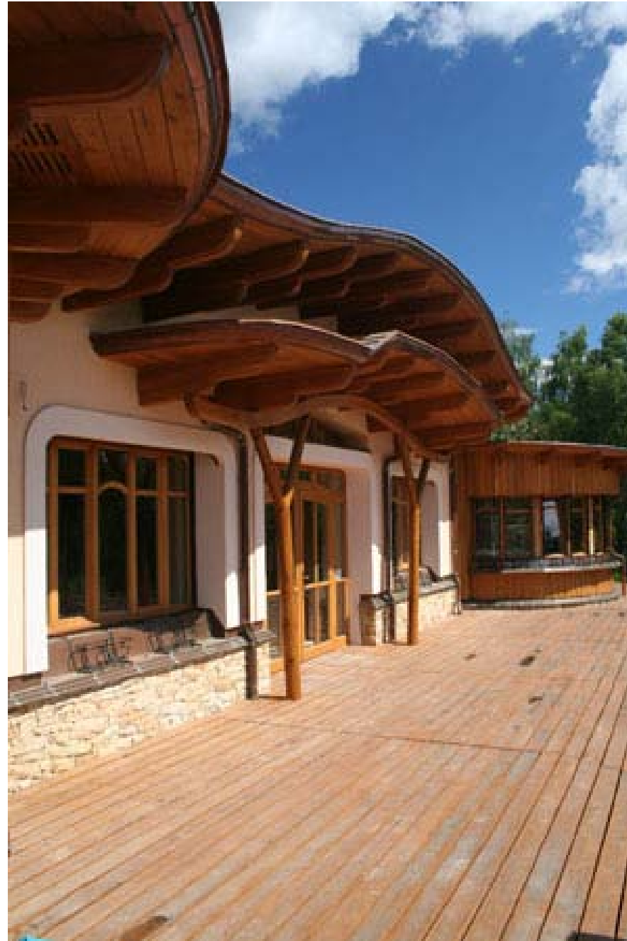
entrance to the outside terrace and garden
