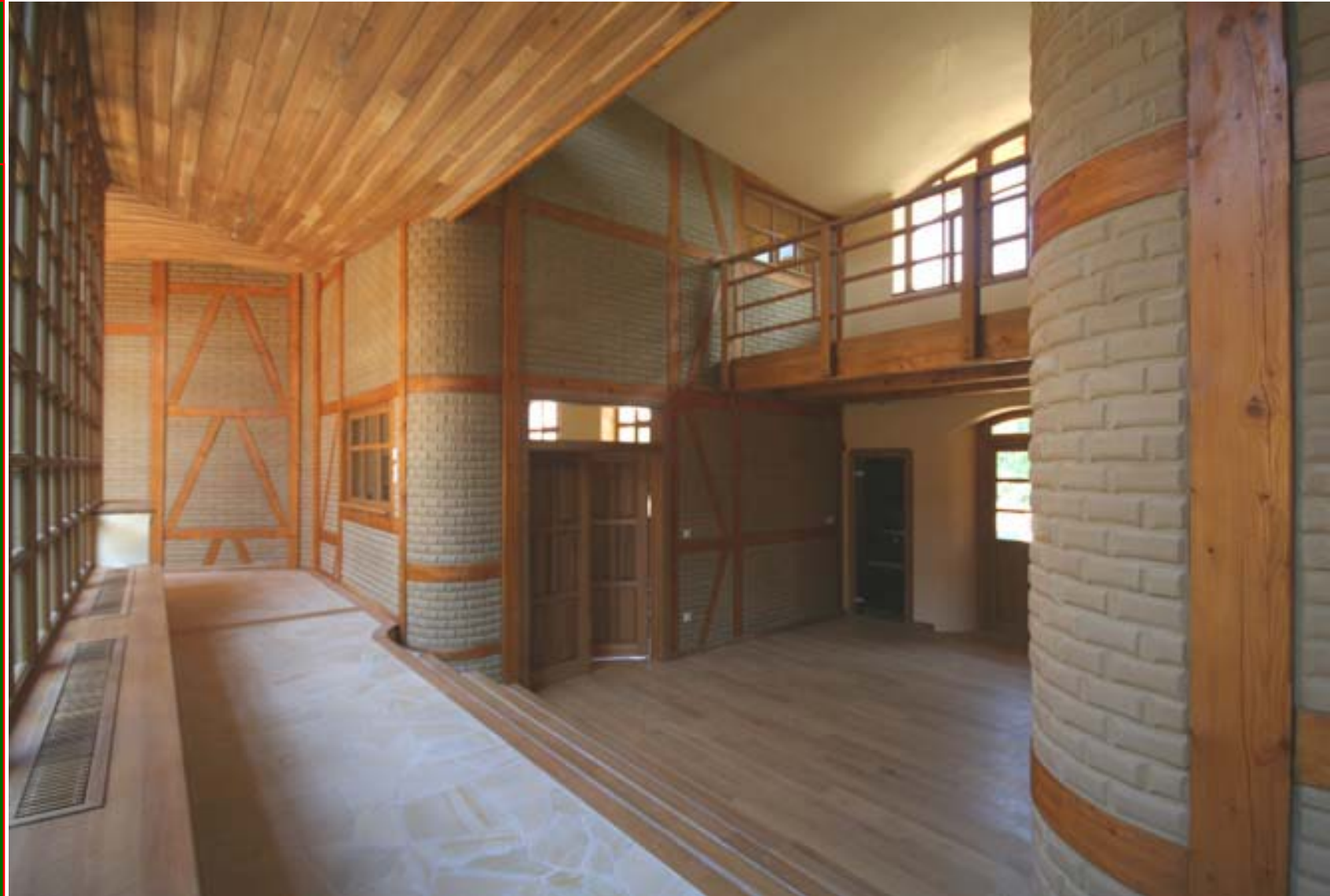
Green roof atrium house, walls in the corridor made of unburnt bricks.
