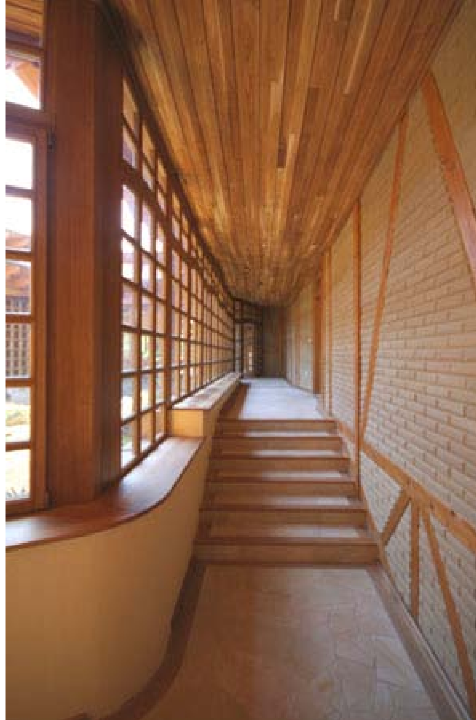
Green roof atrium house, walls in the corridor made of unburnt bricks.
