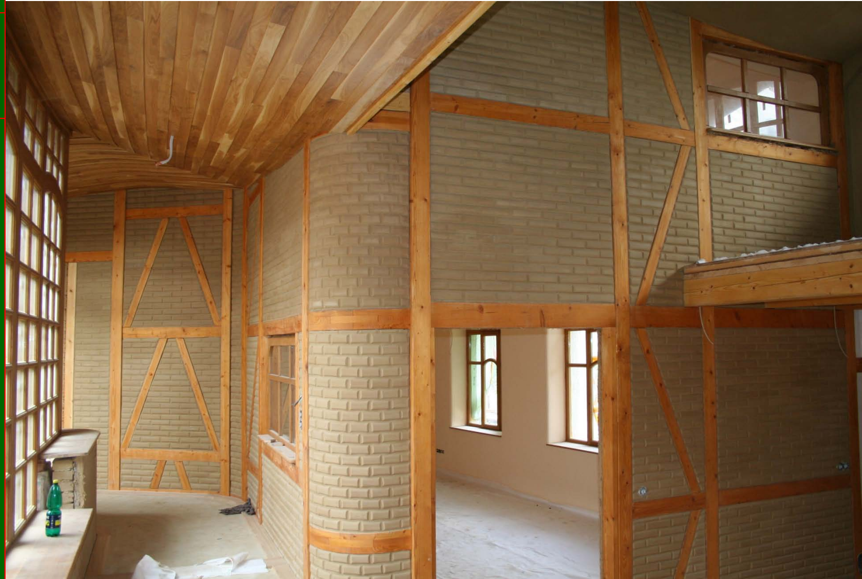
Inside corridor of the house. Walls made of unburnt bricks.
