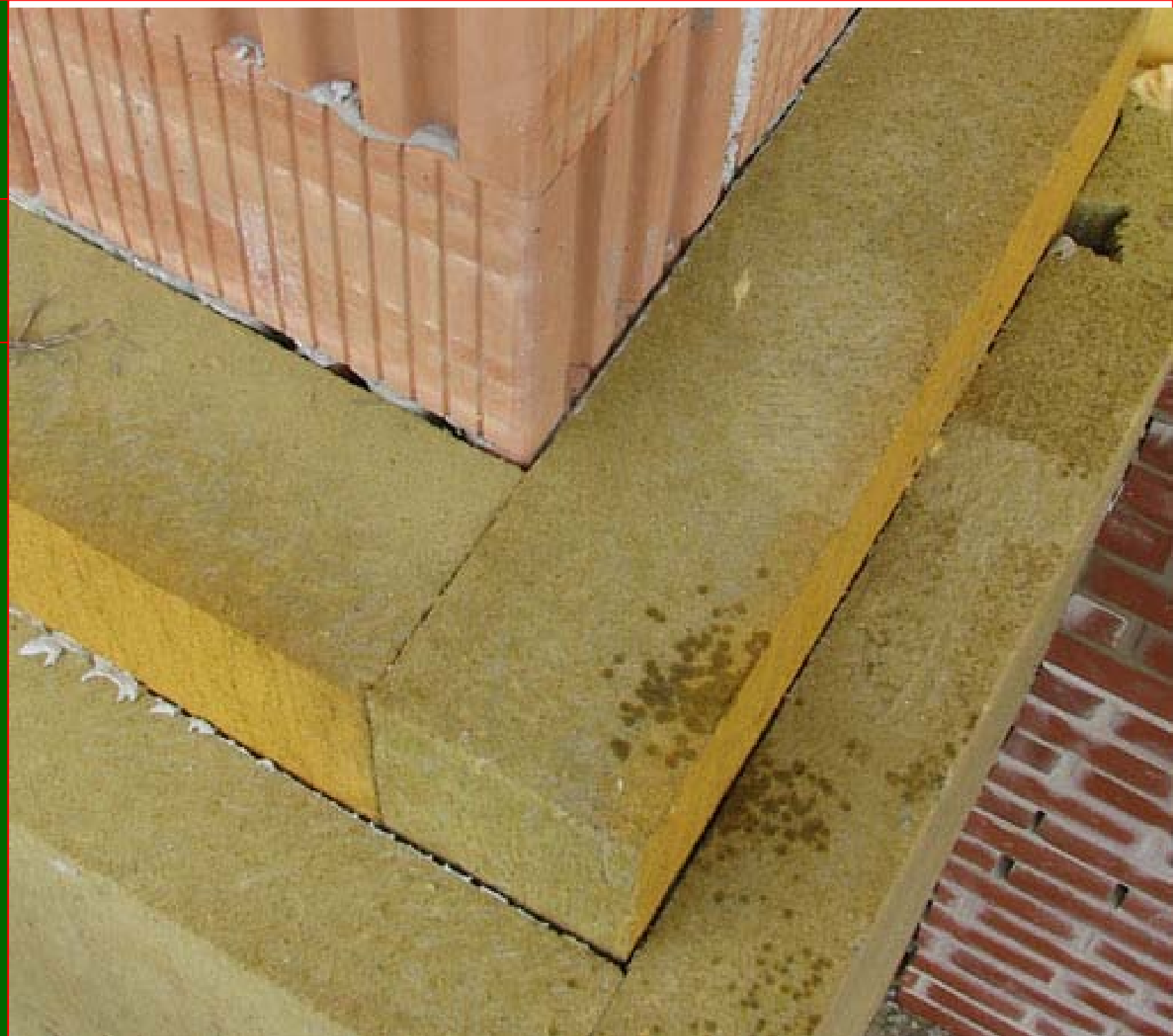
energy efficient house, detail of insulation
