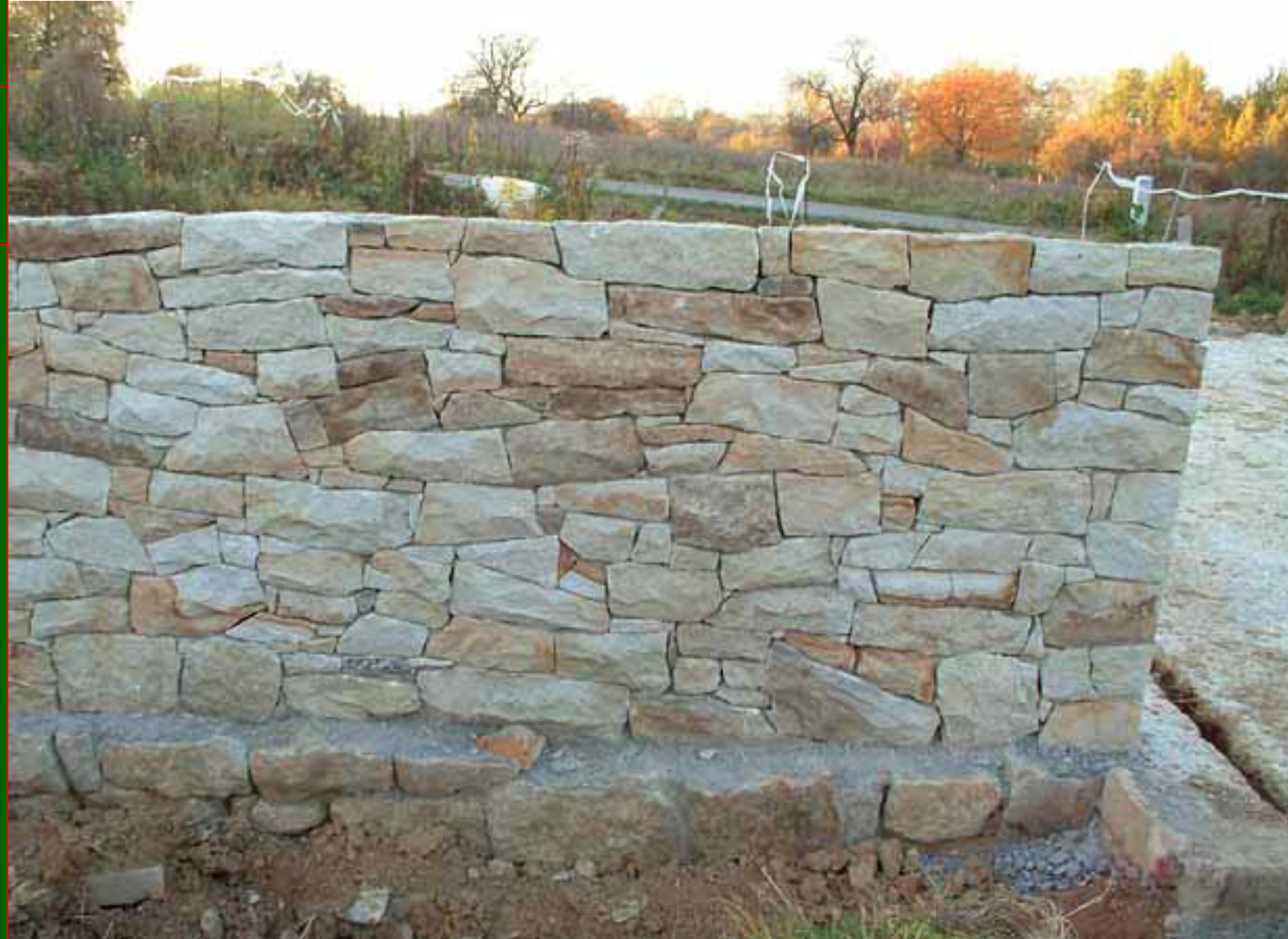
Foundations and base wall made of sand stone.
