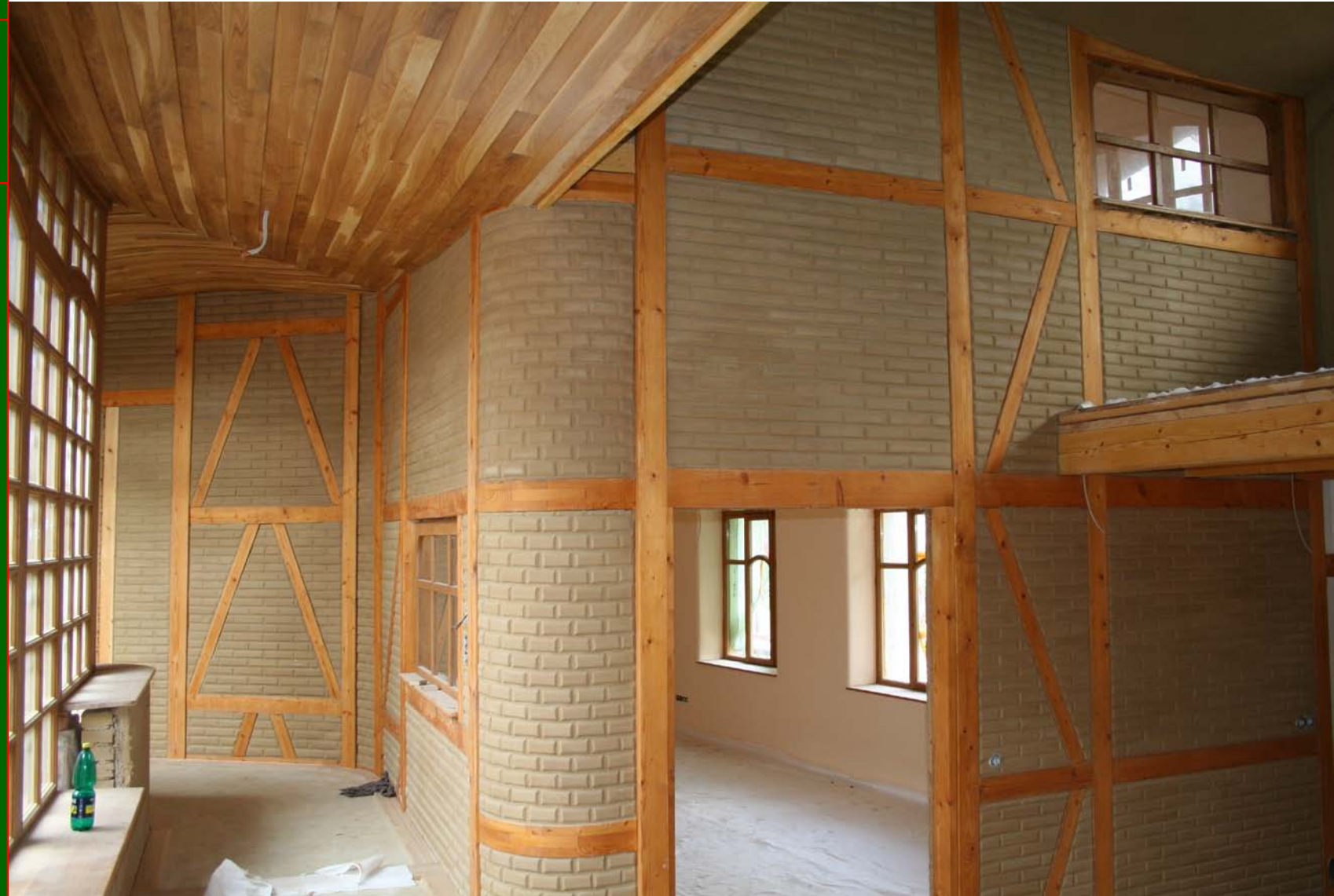
Inside corridor of the house. Walls made of unfired bricks.
